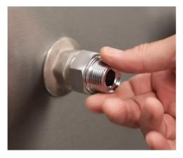
**1** REMOVE existing plumbing fixture. Be sure to KEEP existing hardware connection attached to backsplash. Insert washers and Fisher EZ Install Adapter.
